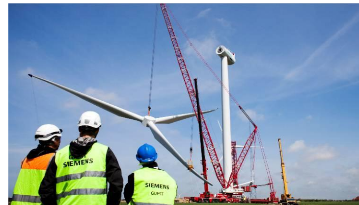
Prototype installation Høvsøre, Denmark
