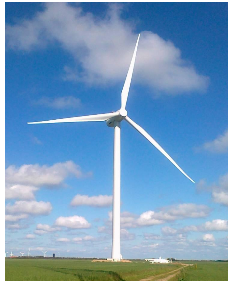
Prototype installation Høvsøre, Denmark
